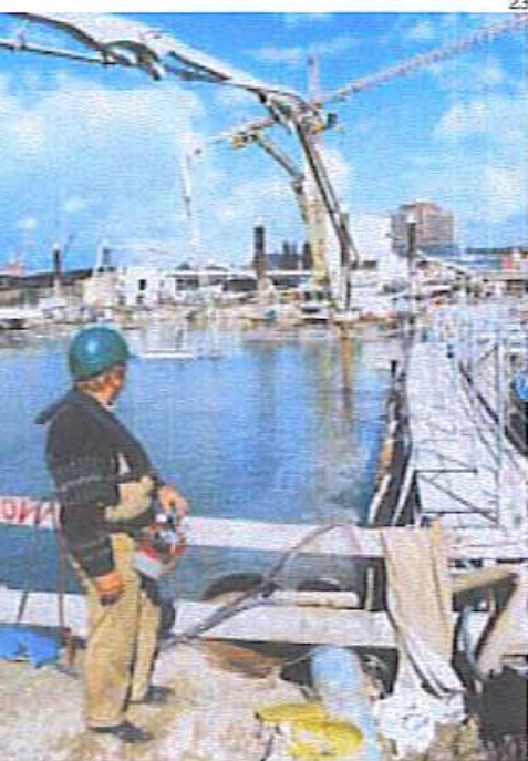
The concrete placing booms are controlled precisely by the ERGONIC radio-remote control
